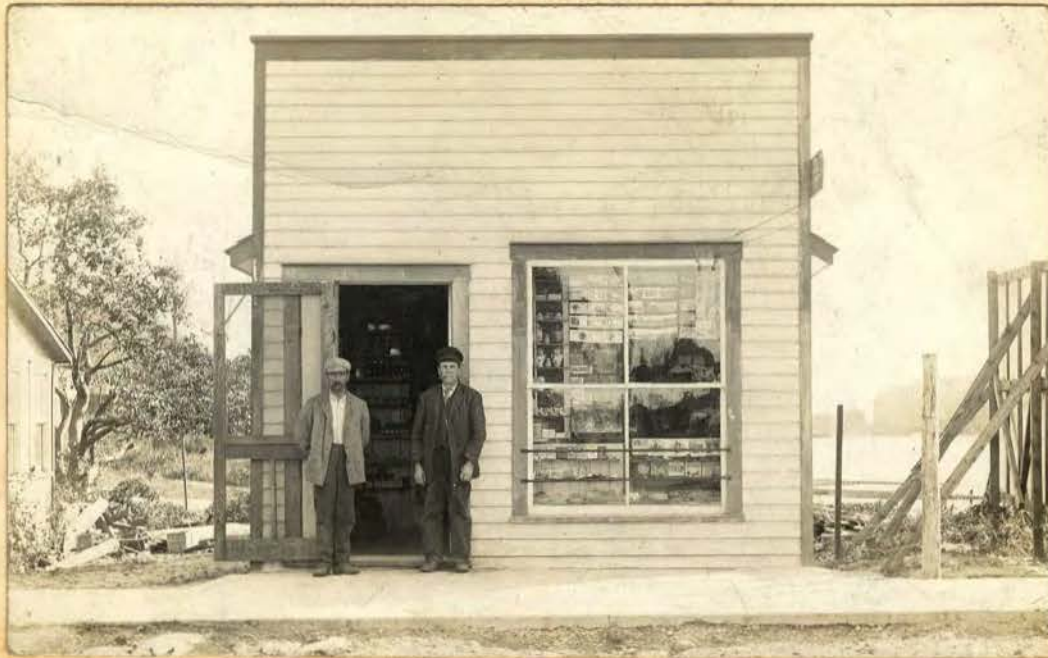
Chas. Hough's Shop-at east of bridge-now -New Library is being erected.
